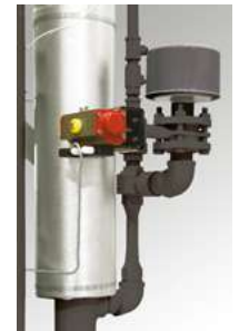
Jet Injection with A 3 Purge Technology™
